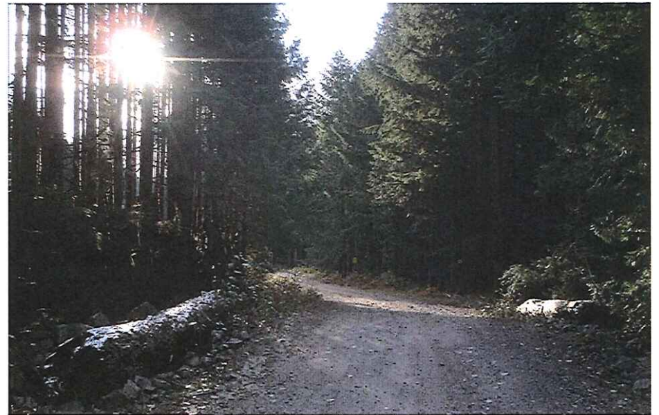
CK2456 Approach Right Bank
